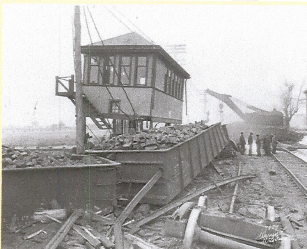
1932 - Big Four Coal Train Pile Up Photo from Ward Suter Collection
